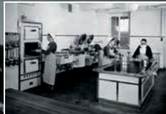
Cooking installation in Kloster 1960
